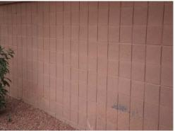
Poor condition. Recommend repair and painting soon. Noted water damage on walls. Includes 8' painted perimeter walls, interior common walls and painted stucco walls surrounding park area. Approx 4800 lf of block walls.
