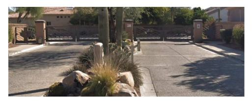
Good condition. 4 metal vehicle gates  $10.5' \times 5.5'$  and 2 metal 7' x 5.5' fence and pedestrian gates.
