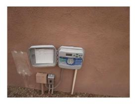
Working condition. (3) Hunter Pro-C 12-station controllers located along walking tract.
