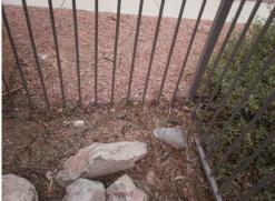
Located at park area. Poor condition. Recommend paint soon to preserve. Approximately 1,400 sq. ft. Some rusting noted. Granite covers the bottom rail in some areas that accelerates rusting of the metal. This component provides a budget for repair in conjunction with painting.
