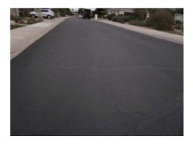
Good condition. Pavement should last indefinitely if maintained on a regular basis. Future updates to this study should continue to evaluate the condition of the pavement and make appropriate adjustments. Approximately 24' wide.
