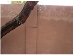
Some wall cracking noted. Recommend repairs be made in conjunction with painting. This component provides a budget for repairs on a 8 year recurring cycle with painting.
