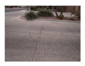
Good condition. Noted some corner cracking. Concrete should last indefinitely.
