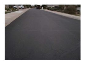
Good condition. Approximately 24' wide. Seal coat applied in 2018. The normal useful life of standard seal coat in Arizona is 3-4 years. Recommend Assn investigate using HA5 (by Holbrook Asphalt) which has a useful life of approximately 7 years. This component budgets for applying HA5 4 years after last seal coat application and then on a 7 year cycle.
