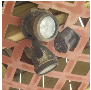
(18) security lights varying types. Some in working condition. Noted some broken or pulling
