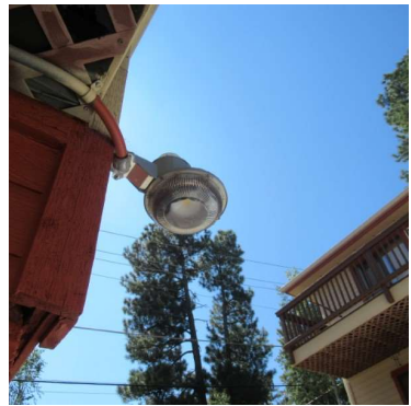
(18) security lights varying types. Some in working condition. Noted some broken or pulling
