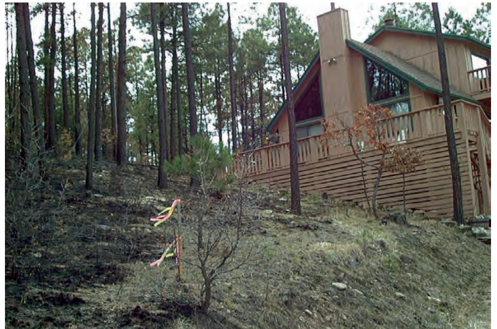
The pre-fire activities implemented by this homeowner include a maintained landscape, use of Firewise plant materials, reduced vegetation around the perimeter of the property and fire-resistant roofing material.
