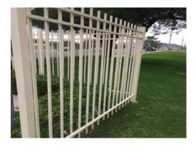
Good condition. Rusting at bottom from irrigation spray. The useful life of this asset has been extended due to its present condition.
