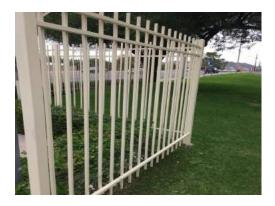
Good condition. Rustining noted on bottom due to irrigation spray. 52' X 6' high wrought iron fence located at entry
