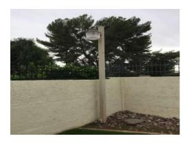
Fair condition. Rusting at bases. Two 10' high metal pole lights. The useful life of this asset has been extended due to its present condition.
