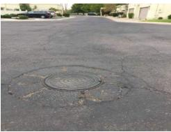
Fair condition. Needs crack seal and repair. Recommend a longer lasting seal coat such as HA5 to be applied next year with a 5 year life and warranty on HA5, slightly more expensive to apply but it has been noted that this propietary product is lasting longer than 5 years.
