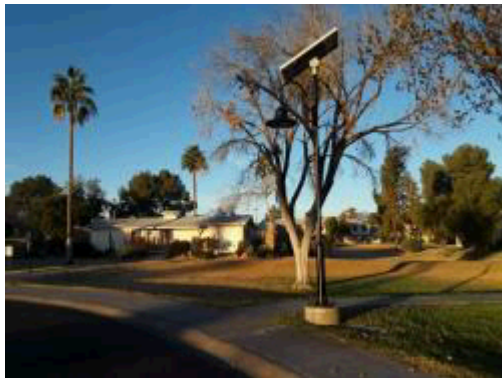
Solar lighting fixtures.
