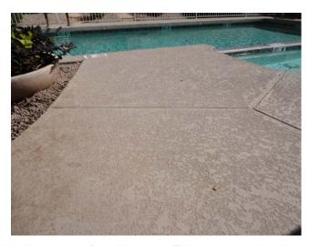
We have estimated that the pool deck was resurfaced in 2011. This component budgets to scrabble & resurface the pool deck on an 18 year cycle. The coating/coloring of the deck following the resurfacing is accounted for in the "Deck - Recoat" component.
