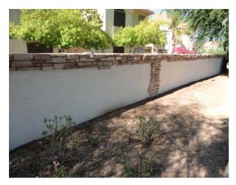
\$1,990 was spent to repaint the stucco site walls (6,280 sq. ft. - west perimeter, north perimeter, trash enclosures, pool equipment enclosure) in June 2014. This component budgets to repaint the stucco site walls every eight (8) years.
