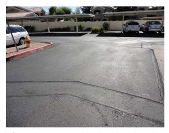
Approximately \$6,500 was spent in September 2014 to crack seal, repair, seal coat & restripe the asphalt. This component budgets for similar work every five years. We have adjusted the cost downward a little bit because we don't anticipate more than \$2,000 in repairs at the time of the next maintenance cycle.
