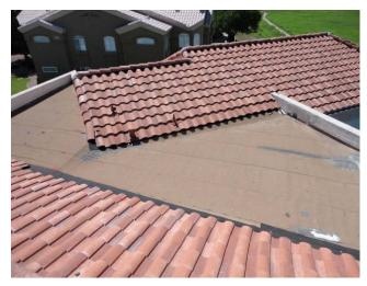
The flat, built-up roof area atop Building D (approx. 425 sq. ft.) will be foamed by Roofing Southwest in August 2017 (\$2,700 fee that has already been paid for with loan proceeds). This new foam roof will come with a 10 year warranty. This component budgets to repair & recoat this foam roof on a continuous 10 year cycle.
