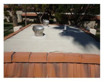
This component budgets to replace the flat, built-up roof w/coating atop the pool building (132 sq. ft.) on a 20 year cycle.
