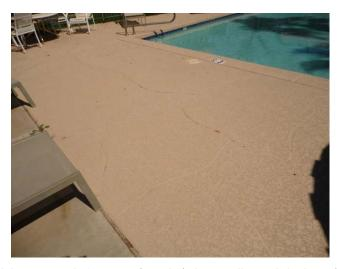
This component includes a provision to repair & recoat (repaint) the acrylic pool deck surface on a six year cycle.
