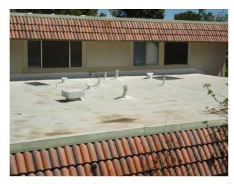
Recoat lower roof (1,300 sq. ft.) on a 10 year cycle. Information & cost provided by Roofing Southwest.
