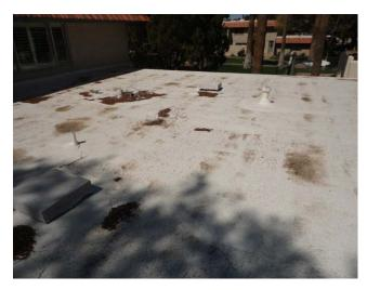
Replace upper roof (2,585 sq. ft.) & lower roof (1,300 sq. ft.) with foam roof - 10 year warranty. Information & cost provided by Roofing Southwest.
