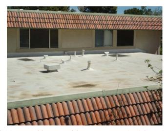
Recoat upper roof (2,585 sq. ft.) & lower roof (1,300 sq. ft.) on a 10 year cycle. Information & cost provided by Roofing Southwest.
