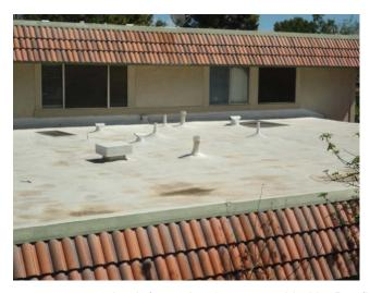
Recoat upper roof (2,585 sq. ft.) on a 10 year cycle. Information & cost provided by Roofing Southwest.
