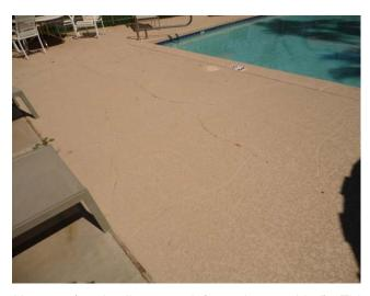
The pool deck was last resurfaced in 2014 (no details or cost information provided). This component budgets to scarify & resurface the acrylic pool deck on an 18 year cycle. The coating/coloring of the deck following the resurfacing is accounted for in the Deck Recoat component.
