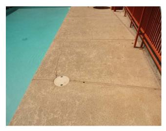
This component includes a provision to resurface the pool deck (includes removal of the existing deck surface and application of new acrylic lace texture overlay). Based on condition, we have scheduled this project for 2020.
