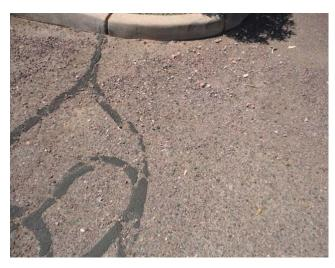
This component includes a provision to pulverize the existing asphalt, removing excess materials, grade and compact pulverized material, and repave with 3" of new asphalt.
