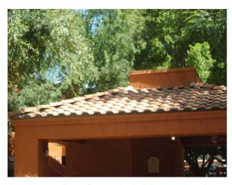
The following comments apply to the concrete tile roofs atop the buildings and pool ramada. Two layers of 40# underlayment were installed during the conversion process.
