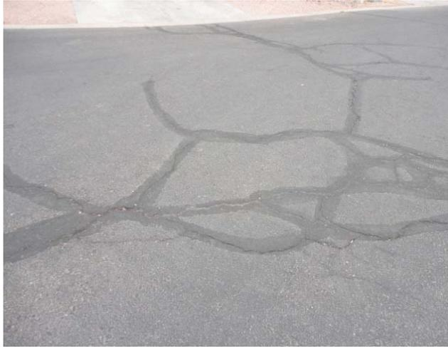
This component includes a provision to repair & seal coat the asphalt making up S. Sharon Court on a continuous five year cycle.
