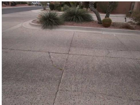
Good condition. Noted some corner cracking. Concrete should last indefinitely.
