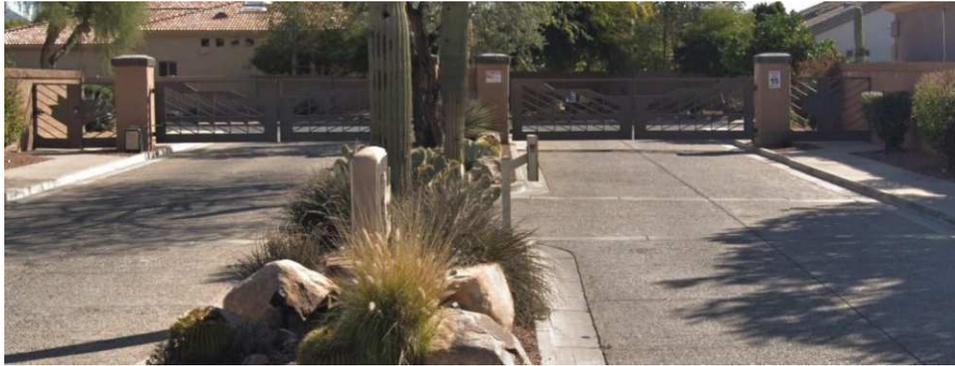
Good condition. 4 metal vehicle gates 10.5' x 5.5' and 2 metal 7' x 5.5' fence and pedestrian gates.
