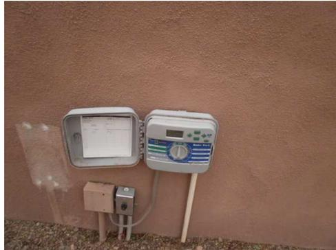
Working condition. (3) Hunter Pro-C 12-station controllers located along walking tract.
