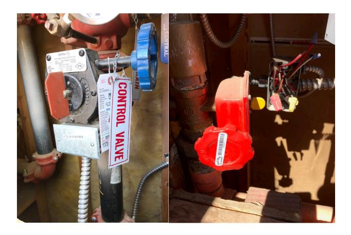
4) Once the control valves are shut and the water is shut off the resident will need to locate the main drain ball valves. The main drain ball valves might have a medal plate that states "Main Drain" and some will not. Once the drain valves are located pull the red or blue handles which will release the water & pressure from the sprinkler system. There might be two drain valves or three drain valves depending on how many floors the building has. Make sure to open the drain valves all the way.
