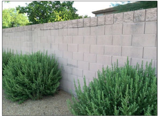
CMU Wall Repair Paint
