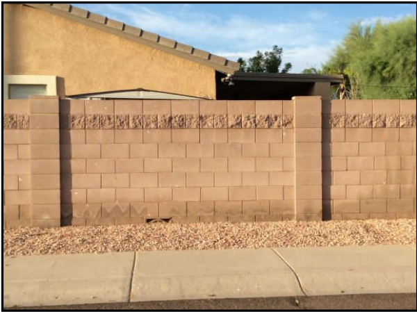
CMU Wall Repair Paint
