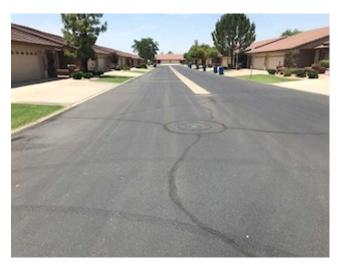
Holbrook Asphalt seal cracks in July 2016 for \$1,712. We have used this cost as a basis and have scheduled ongoing crack seal every four (4) years.
