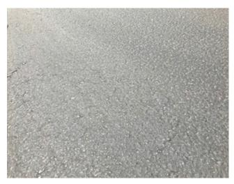
Holbrook Asphalt completed a project to apply an HA5, High Density Mineral Bond asphalt preservation treatment to the community asphalt in July 2016 for \$16,244.98, including repairs and crack sealing. This product comes with a five (5) year manufacturer and contractor warranty, but should last 7 - 8 years before re-application is necessary. Therefore, we have used an eight (8) year useful life.
