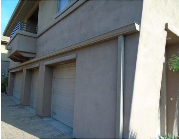
The aluminum gutters & downspouts have an indefinite life if maintained properly and cleaned out on a regular basis. Good maintenance practice won't allow the need to accumulate reserves to a point of major expense. Minor repairs & clean outs should be handled on an "as needed" basis using operating funds.
