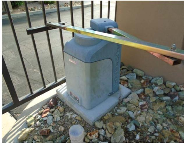
These are LiftMaster, CSW24V, swing gate operators with February 2014 manufactured dates on the exit side.
