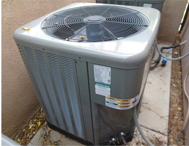
Rheem, 5 ton split system w/heat pump (replaced in late 2018 at a cost of \$6,736.00).
