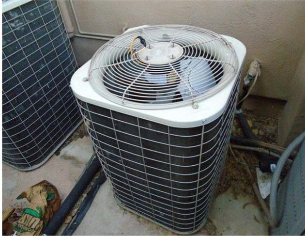
This is a Bryant, 2.5 ton split system. As requested by the client, we are budgeting to replace this system by 2020, due to the discontinued use of the R-22 freon by 2020.
