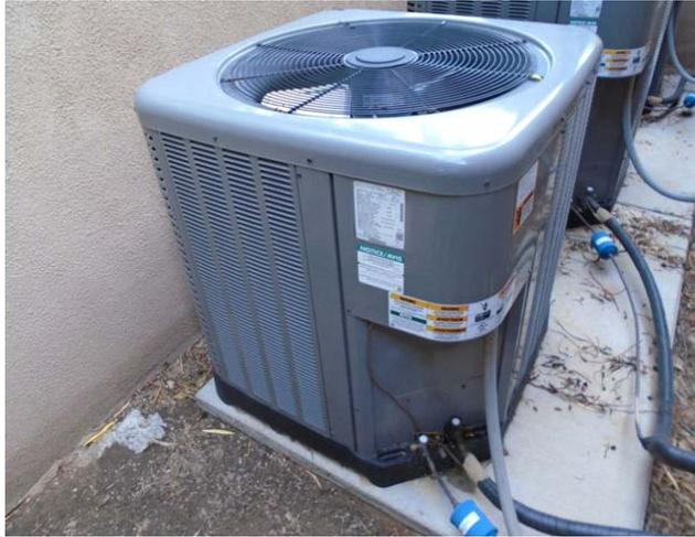
Rheem, 3.5 ton split system w/heat pump (replaced in late 2018 at a cost of \$6,528.00).
