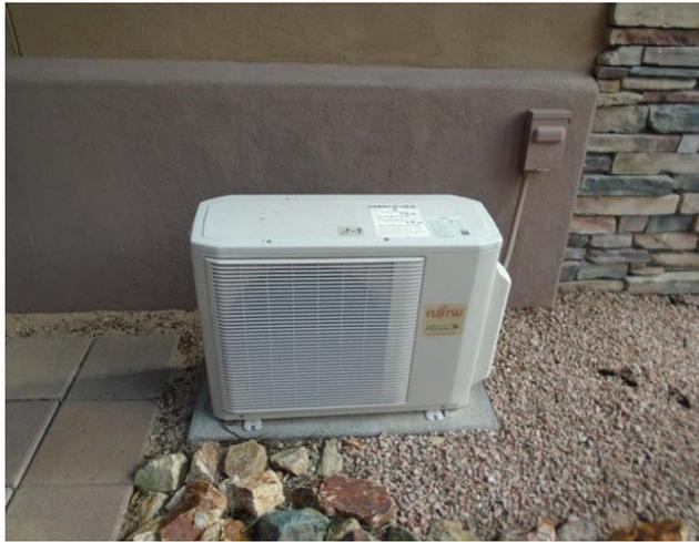
This is a Fujitsu, 1.5 ton mini-split, ductless HVAC system.
