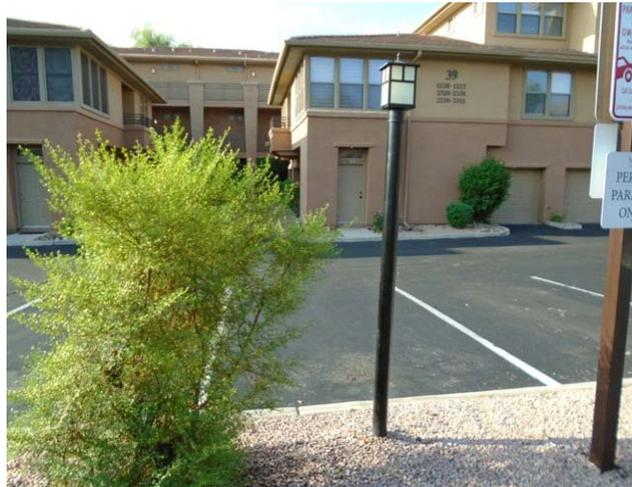
There are 45, pole mounted lantern fixtures scattered throughout the community. \$10,909 was spent in August/September 2017 to upgrade/replace the fixtures with LED fixtures. We have used a 25 year useful life cycle going forward. The cost used also includes a provision for metal pole replacements on an "as needed" basis.
