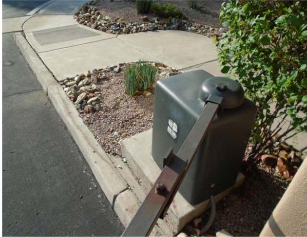
These are Elite, CSW200ULDC3, swing gate operators with October 2006 manufactured dates on the entrance side.
