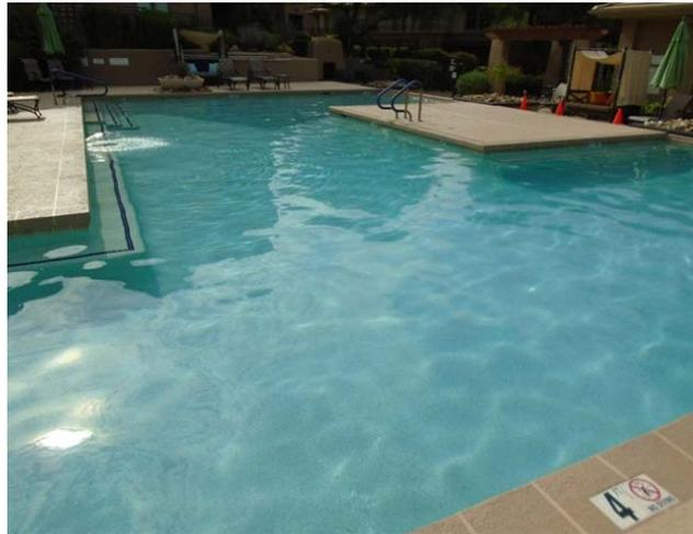
The pool (3,100 sq. ft internal area) was resurfaced with white mini-pebble & retiled (252 LF of trim tile, 170 LF of bench tile) in May 2015 at a cost of \$24,025. Going forward, this component also includes a provision to replace the wall mounted ceramic tile at the water features (+/- 126 sq., ft.) on an "as needed" basis.
