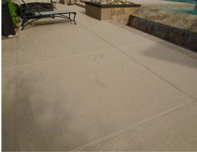
The front pool acrylic deck surface was machine stripped and resurfaced in September 2014 at a cost of \$41,933.79, and again in August 2020 at a cost of \$39,235. This component budgets for similar work every nine (9) years. The coating/coloring of the deck following the resurfacing is accounted for in the "Deck Recoat" component.
