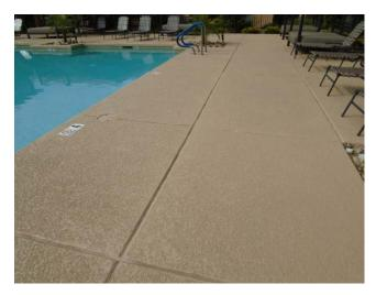
This component budgets to machine strip & resurface the acrylic deck on a 15 year cycle. The coating/coloring of the deck following the resurfacing is accounted for in the "Deck Recoat" component.
