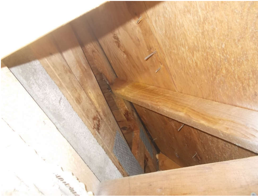
Photo 1: View of typical mansard framing at north/south sides of units. Connections do not have appropriate framing hardware. MODIFICATIONS ARE REQUIRED.
