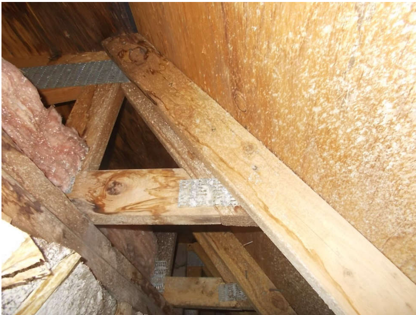
Photo 2: View of typical mansard framing at east/west sides of units. Mansard framing is "sistered" to side of roof trusses and appears to be stable and code compliant. NO MODIFICATIONS REQUIRED.
