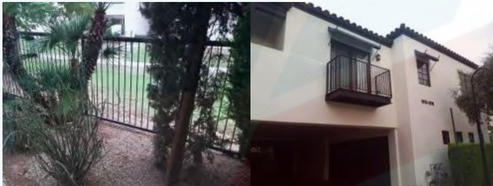
Pole Lights ($5000), Pool Fence ($2000), Balcony Rails & Decks ($8000)
