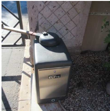
Working condition. Chamberlain Elite swing arm operators with mfg date 2012.
