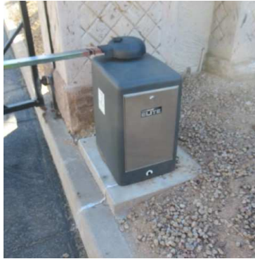
Working condition. Chamberlain Elite swing arm operators with mfg date 2009.
