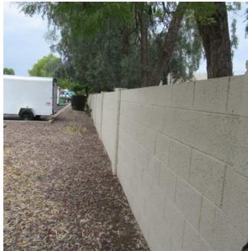
North wall leaning due to trees on commercial property. It is a 4" dually wall with what appears to be very little foundation. West wall chipped due to landscape irrigation. South wall against alley in poor condition. East perimeter wall patched along tract C. Block degrading.
