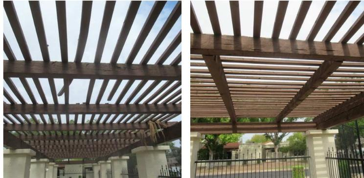
Poor condition. Noted popping slats, broken slats, wood disintegrating, etc. Approximate pricing is between \$10-\$14, used middle for the study.
