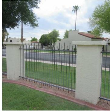
Fair to poor condition. Noted significant rusting. Budget assumes that repairs includes painting of the new fence.
