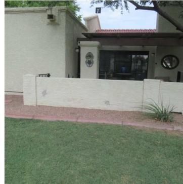
Showing numerous stucco repairs, paint poor chipped. Mold on unit 29. To coincide with community paint asset ID 1024.
