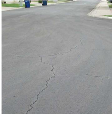
Includes Sunburst Lane, Krista Way and Taylor Drive north of Louis Way. Pavement was replaced in 2012. Pavement is in good condition with block cracking present.
