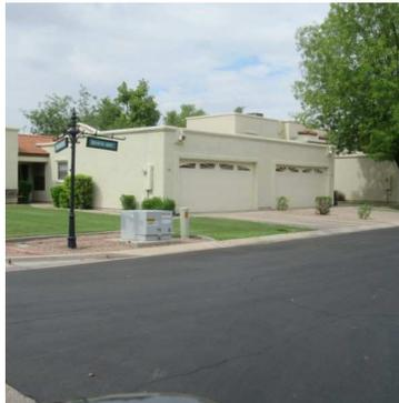
Good condition. Normal asphalt cracking noted. Seal coat and crack seal done in 2021. Recommend seal coat and crack seal on regular basis.
