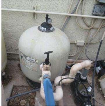
Working condition. No leaks noted. Pentair Triton II TR-60, 3.14 sq. ft sand filter.
