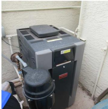
Working condition. Raypak 266K BTU gas heater. Model C-R206A-EP-C ASME.
