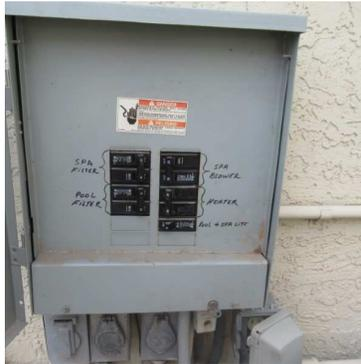
Good condition. 125 amp panel located in covered pool equipment area. Anticipate it is original install.
