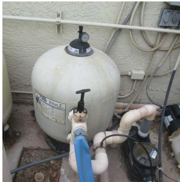
Working condition. Pentair Triton II TR-100, 4.91 sq. ft. sand filter.
