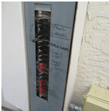
Older condition. 200 amp panel located on pool building. It is exposed to sun and weather elements. Anticipate that it is original equipment.
