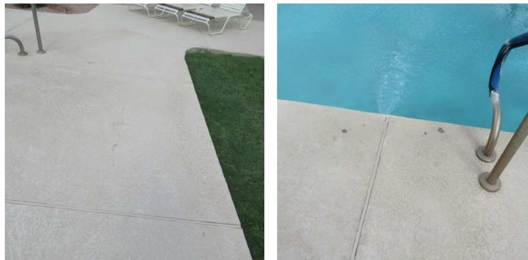
Poor condition. Noted chipping and cracking. Repairs in 2017 for approximately \$10,000.
