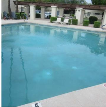
Poor condition. Noted fading, tile older condition. Recommend resurface in 2023 to preserve.
