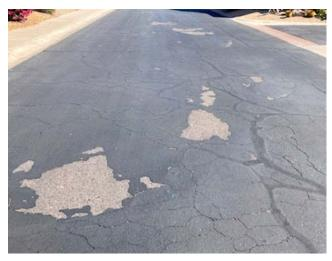
Holbrook Asphalt completed a project to install HA5 High Density Mineral Bond in 3/2017 for \$19,778.58. We are budgeting to reapply in 2024 per the current proposal from Holbrook Asphalt of \$34,063.11. Per Terri Troy, add a 5% - 10% increase in the event that the work can't be completed for several months.
