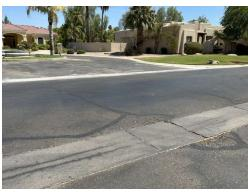
The pavement is generally in good structural condition. There is some alligator cracking but is a very small percentage of the total pavement. Some repairs should be anticipated in the future if the blocks of asphalt in the alligator crack areas begin to move or break-up. The pavement should be maintained with a good surface treatment and cracks sealed on a regular basis. With a good maintenance program the pavement should last several more years.
