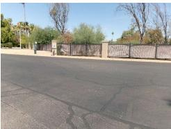
Budget for elastomere crack repair from Holbrook bid in 2023. Cracks should be sealed on a regular basis normally on a three cycle.
