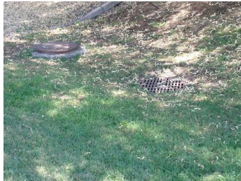
Dual chamber drywells. Drywells are recommended to be inspected and cleaned every 3-5 years.
