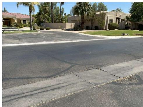
The pavement is generally in good structural condition. There is some alligator cracking but is a very small percentage of the total pavement. Some repairs should be anticipated in the future if the blocks of asphalt in the alligator crack areas begin to move or break-up. The pavement should be maintained with a good surface treatment and cracks sealed on a regular basis. With a good maintenance program the pavement should last several more years.
