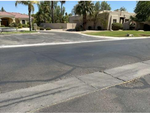
The pavement is generally in good structural condition. There is some alligator cracking but is a very small percentage of the total pavement. Some repairs should be anticipated in the future if the blocks of asphalt in the alligator crack areas begin to move or break-up. The pavement should be maintained with a good surface treatment and cracks sealed on a regular basis. With a good maintenance program the pavement should last sevmore years.
