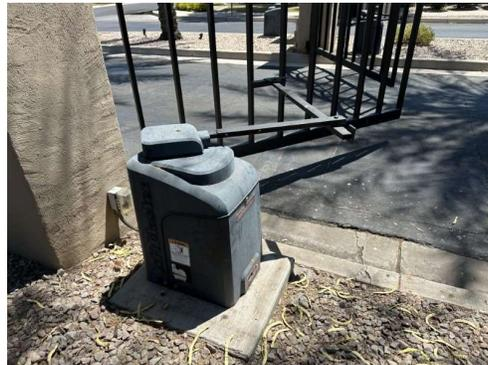
(4) Liftmaster CSW24VDC, swing gate operators. Mfg date 5/2015.
