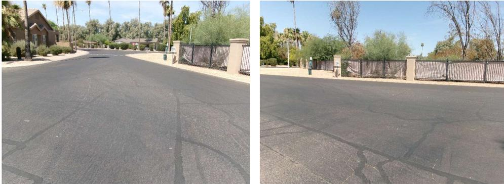
Budget for elastomere crack repair from Holbrook bid in 2023. Cracks should be sealed on a regular basis normally on a three cycle.
