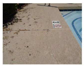
This component includes a provision to resurface the pool deck (includes removal of the existing deck surface and application of new acrylic lace texture overlay).
