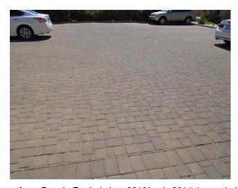
Based on historical satellite images from Google Earth, in late 2013/early 2014 the asphalt was removed and replaced with concrete pavers. This component will accumulate funds for repairs to these pavers ever 15 years. No provision for complete replacement has been included in this analysis.
