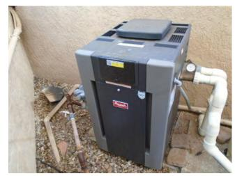
This is a RayPak, 266,000 BTU input heater (installed in early 2023 per the client).
