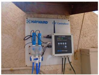
This is a CAT 4000 chemical automation system. We have adjusted the useful life because this system was repaired in early 2023.
