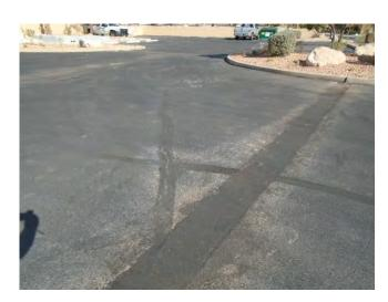
The parking lot asphalt was crack sealed, seal coated & restriped in mid-2022 by Bates Paving & Sealing, Inc. at a cost of \$6,527. This component budgets for similar work every five (5) years, and also includes a provision for asphalt repairs.
