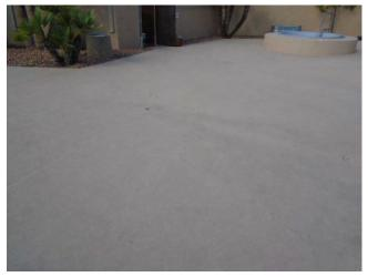
In August 2023, the client received a bid from E-Konomy Pool Service & Supplies to scarify the acrylic deck surface (11,000 sq. ft.), fill cracks, retexture the deck, and coat with two coats of sealer and restorer at a cost of \$104,500. This work is not currently needed, but has been scheduled to occur in 2031, and then on an 18 year cycle.
