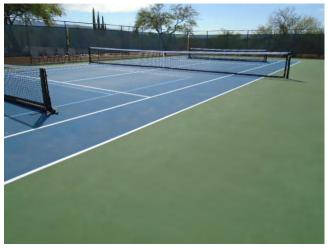
The two tennis courts were crack filled, resurfaced & restriped in mid-2022 by Outplay Sports Surfacing at a cost of \$15,400. The client has advised us to budget for similar work every four (4) years.
