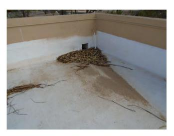
The flat, built-up roofs atop the clubhouse & pool area ramada were coated/recoated in mid-2022. This component budgets to coat/recoat these roofs on a five (5) year cycle.
