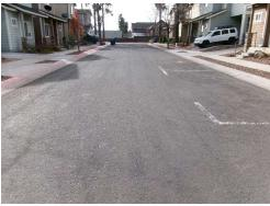
Structurally good condition. Limited cracking. Appears that a slurry seal had been applied at some point. Recommend surface treatment and crack seal soon to preserve. Unknown year of last surface treatment.
