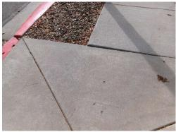
Good to fair condition. Sidewalks, curbs and intersection paving. Noted cracking and lifting of sidewalk. Landscaper noted grind areas that are continually moving forward.
