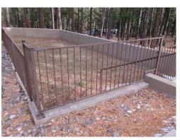
Good condition. Metal fence on border of two retention basins. Approximatley 460 LF.
