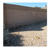
Poor condition. Faded and cracking. Recommend painting soon. Last painted in 2008 for \$13,697. Some block walls and view fence in hard to access areas due to terrain and vegetation. Masonry walls painting to coincide with metal painting see asset ID 1006.
