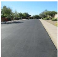
Good condition. HA5 applied by Holbrook Asphalt Co. on 8/3/2018 for a total of \$30,269. HA5 has 5 year warranty so set useful life at 6 years. Life adjustment due to Pinnacle Paving applying PMM 6/2019 over a paint spill paid for by City of Scottsdale.
