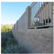
Fair to good condition. Rust visible in some locations. Includes: (4) entry/exit gates, (3) pedestrian gates, fencing along south perimeter next to lot 32, fencing at the ends of cul-de-sacs on west perimeter, view fencing along boundry lines between lots and common areas and caps at pedestrian gates. Approximately 7,760 LF of fencing. Last painted by Advanced Painting & Contracting in 3/16 for \$38,304.
