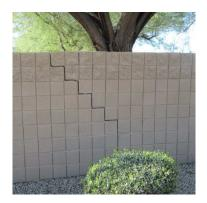
Good condition. Noted the cracks have continued to open up since prior study. Noted some cracking due to trees and irrigation overspray. This asset is for metal fencing and masonry wall
