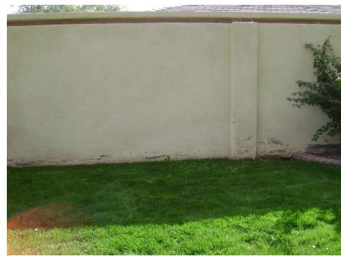
Poor condition. Budget to paint masonry block stucco walls. Locations include entrance,
