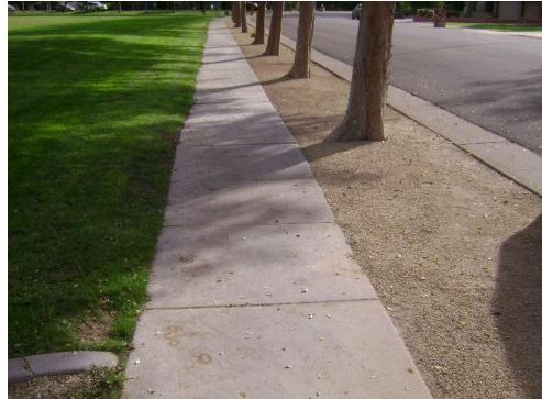
Fair condition. Budget to repair and/or replace sections of concrete walkways or landscape curbing when needed. Noted lifting of sidewalk due to tree roots.
