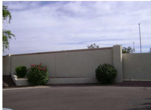
Various conditions. Budget to repair painted stucco walls. Location along Price Rd. Recommend paint with minor stucco repair soon to preserve and aesthetics. In conjunction with wall paint, see asset ID 1008. Approximately 17,000 SF of wall.
