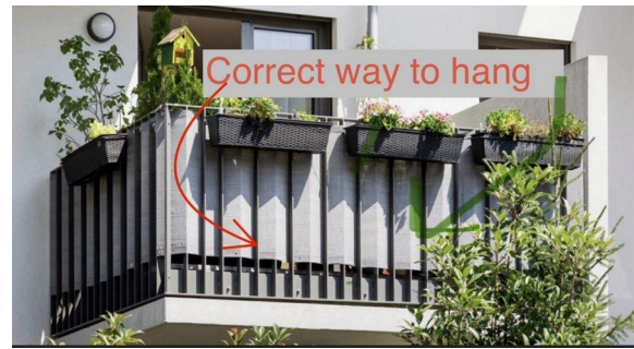
✓ CORRECT — hung inside the railing
