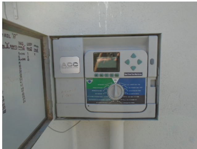
This is a Hunter ACC-99D controller located at the entrance to the community.
