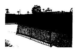
Block walls are in good condition. Normal useful life of block walls is 35 years. Based on the age of the community these walls are probably 30+ years old. Based on the condition it is estimated that these walls should last another 30 years with some repair. This study estimates that 10% of the wall will need replacement in 30 years.
