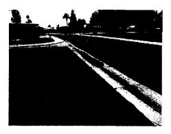
The concrete curb and sidewalks are in good condition with few signs of structural failure. These should last indefinitely. No replacement is scheduled. Small damaged areas may need to be replaced from maintenance funds.
