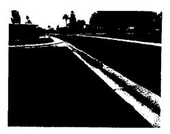
The pavement has multiple cracking probably resulting from exposure to UV and normal wear. Normal life for asphalt pavement is 20-30 years. This pavement if placed in the mid 70's is approaching 40 years. Some areas should be replaced due to structural failure. Repairing select areas and sealing could extend the life of the pavement 20+ years.
