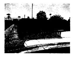
Fence is in good condition and should last several years if paint is kept in good condition.
