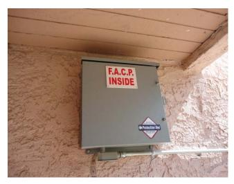
Each of the five buildings has a fire alarm control panel and associated components. The age of each panel varies, and no historical installation/replacement information was provided by the client. This component will accumulate \$3,000, every five years, for replacements associated with the fire alarm control panels and associated components on an "as needed" basis.
