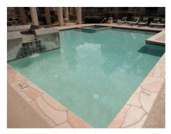
We have estimated that the pool & spa were resurfaced (pebble) & retiled in 2010. This component budgets for similar work on a 25 year cycle. However, the accumulated funds should be used on an "as needed" basis to replace the tile more frequently, if necessary.
