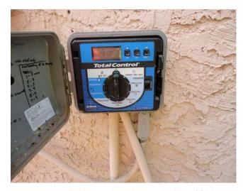
This is an Irritrol Total Control, 12 station controller located on the north side of Bldg 5.
