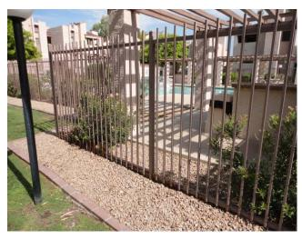
The age of the wrought iron fencing & gates at the pool area is unkown. However, it does not appear to be the original fencing. For budgeting purposes we have used 2004 as the basis for aging it. The pool fencing is severely rusted in multiple locations, and unsteady in a couple locations. This component includes a provision to replace the following pool area wrought iron on a 20 year cycle.
