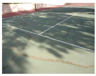
The asphalt tennis court is in poor condition (significant cracking), and has been for quite some time. We do not know the client's intentions concerning the tennis court and related components (chain link & lighting). Therefore, this component includes a provision to install a post-tension concrete court in 2024.
