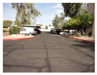
Other than the repair & seal coat project completed in 2016, the client was unable to provide any other historical asphalt maintenance information. However, it does appear as though a slurry seal was applied at some point in the past. Currently, the asphalt is showing its age with significant cracking and several areas where repairs are needed. Overall, the asphalt is nearing the end of its useful life.
