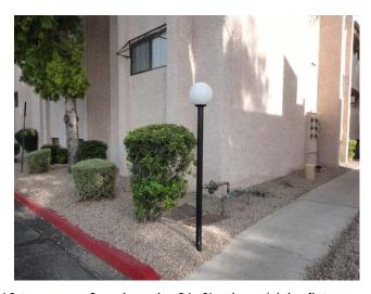
\$5,612.12 was spent in April 2016 to remove & replace the 21, 6' poles w/globe fixtures scattered throughout the community. The cost included new concrete footings (12" x 12"), new electrical wires installed up the poles, and LED bulbs. This component budgets for similar work every 30 years.
