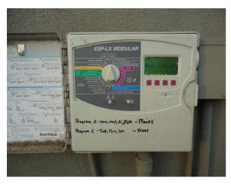
This is a Rain Bird ESP-LX modular controller with 24 stations, located at the trash enclosure. We have estimated when it was replaced.
