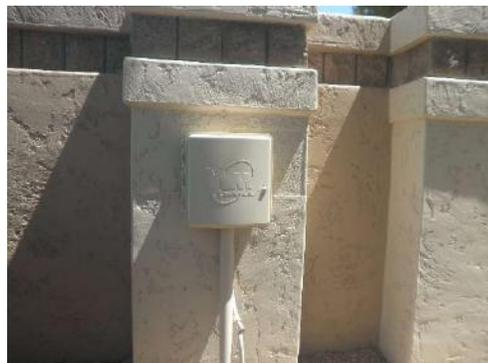
(1) 36 station Weathermatic SL4800 Smart Timers irrigation controller @ Saddle Park & (1)
