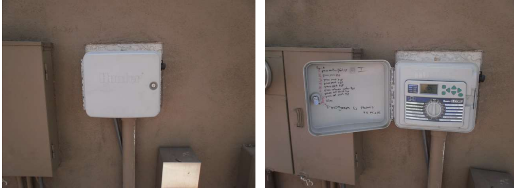
1 Hunter I-Core model IC-600-PL. 10-station used on a 27-station controller.
